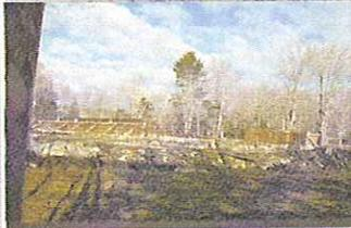
After the site was cleared, it was time for the foundation to be poured. This photo, taken on **April 6th**, shows the framework for the concrete to be poured into.
