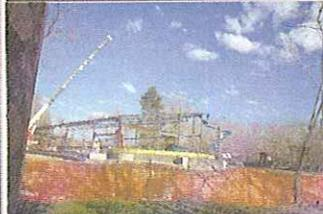
After the foundation was poured, it was time for the frame to be put up! This photo, taken on **May 9th**, shows the crane moving the beams into place.
